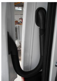
ELECTRICS CABLED THROUGH DOOR
